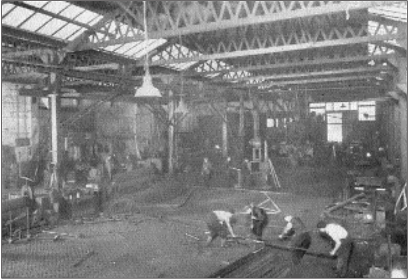
A section of the plating shop.
